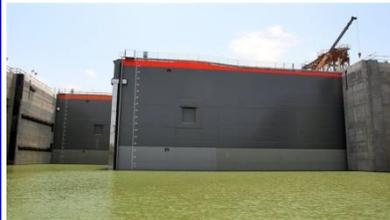
A lock is a hydraulic structure to make it navigable channel and allow boats to negotiate height differences. The lock comprises a lock in which it is possible to vary the level of water and is delimited by the doors. The locks of the Panama Canal aim maintenance of pools, without traffic interruption.
